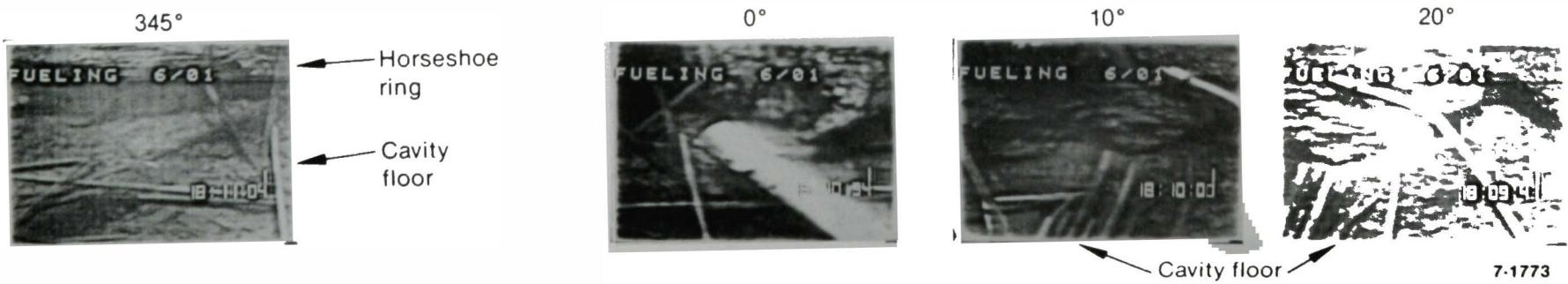
Plate A-6A. Horseshoe ring between 335° and 25° azimuth (North) before (06/01) and after (10/12) core boring.
