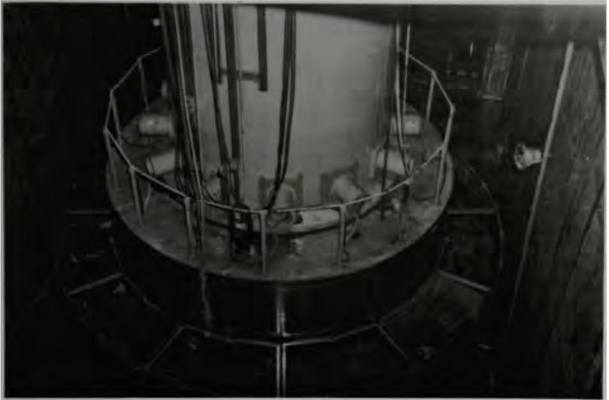
Figure 9. View into the transfer canal—July entry. The shield tanks around the vessel head are dry.
