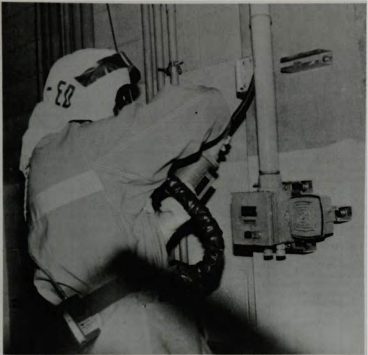
Figure 2. Removal of the HP-RT-211 radiation detector.
