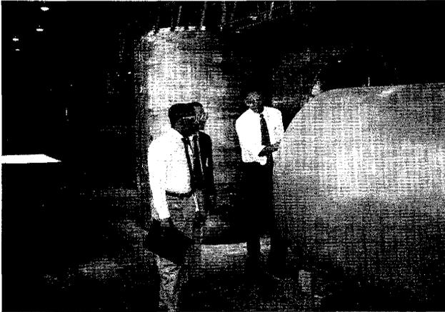
NMSS Inspector (from left) D. Reid, K. Leu, and S. O'Connor perform safety inspection of the primary containment vessel of the VSC-24 dry spent fuel storage system.
