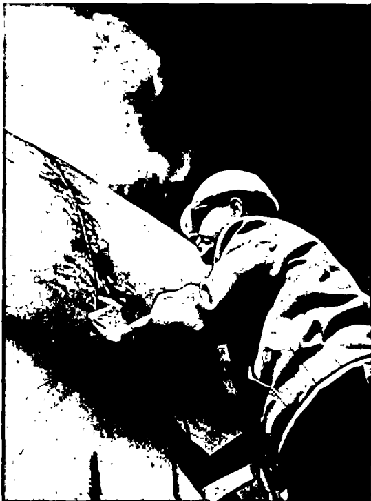
NRC standards, regulations and guides serve as bases for inspections by field inspectors throughout the lifetime of a nuclear reactor, and all safety related components must meet rigid quality assurance criteria. Here, an NRC inspector checks welding on a process water tank dome.
