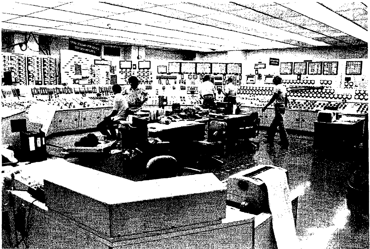
The control room for TMI Unit 2 is shown above. The instruments and controls are deployed in a U-shaped pattern in a design intended to permit one operator to supervise operations under nor-
