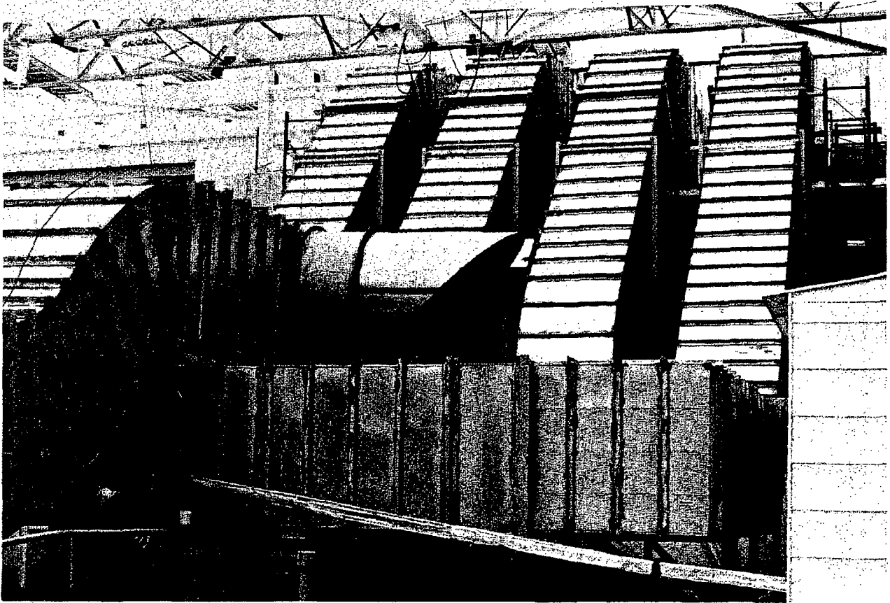
A new ventilation filtration system was installed on top of the auxiliary building of Unit 2 when the NRC determined that the existing system was not functioning satisfactorily after the accident.
