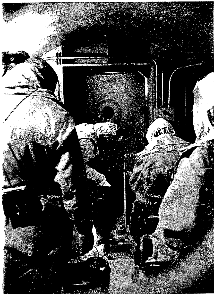
A milestone in the post-accident cleanup at TMI-2 was reached on July 23, 1980, with the first entry into the reactor building since the accident on March 28, 1979. The licensee's personnel are shown in protective clothing with communications and radiation detection equipment as they prepare to enter the inner door of the personnel access hatch.
